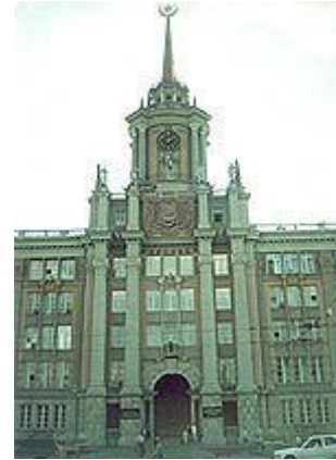
City Council, Ekaterinburg (1947-1954) - built on the place of the Cathedral Temple (demolished in 1930), it looks right in the eyes of bronze Lenin statue.
