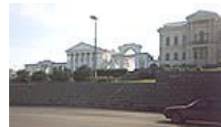
Palace of Merchant Rastorguev (1794-1795) , Vosnesenskaya Hill, Lunacharskogo Street. In 1935-1937 the palace was reconstructed and became the Palace of Pioneers - the recreational center and school of arts for children.
